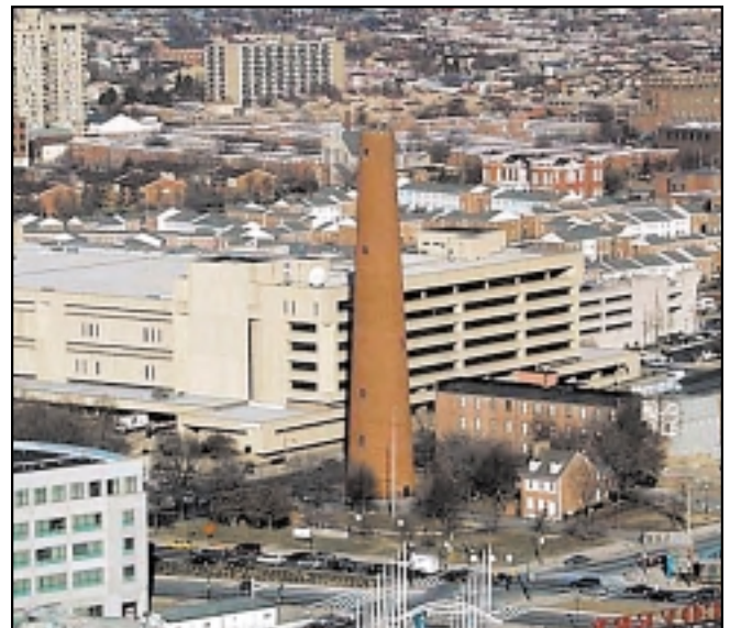
Shot Tower, a National Historic Landmark in Baltimore's Inner Harbor. From 1828-1892, molten lead was dropped from the top of this 234 foot tower through a sieve and into a vat of water to form lead spheres to be used as rifle shot. Photo courtesy of www.baltimore.to .
